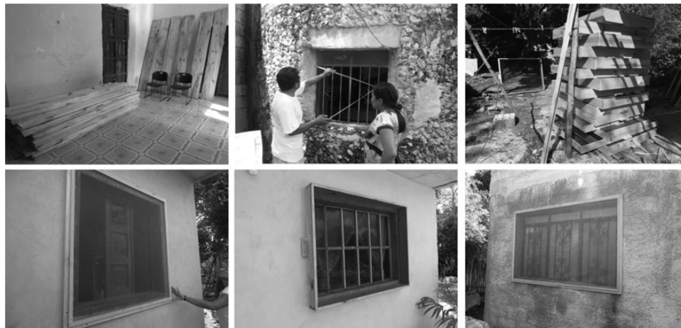
Figure 3. Manufacture and installation of insect screens for vector control. All screens were manufactured locally in the communities, using a high-quality fiber mesh with a wooden frame fitted to each bedroom window.
